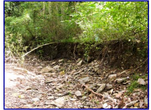
RC2 will help Lyn Farrel address erosion issues in Cedar Creek (Anna Bourke)
